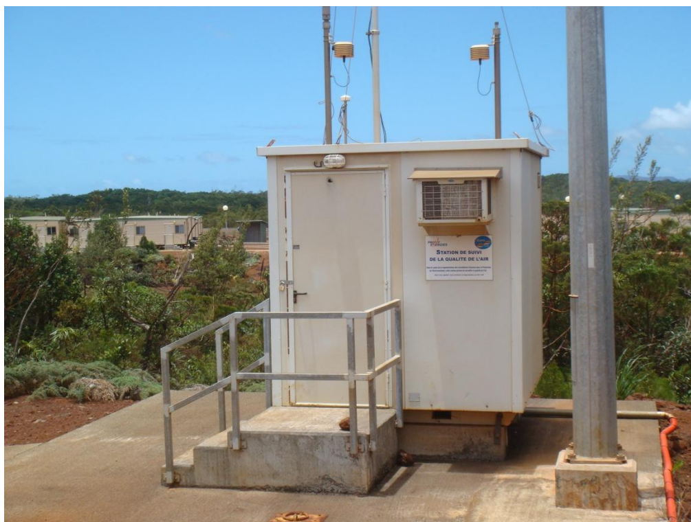
Figure 4: Station de la Base Vie
