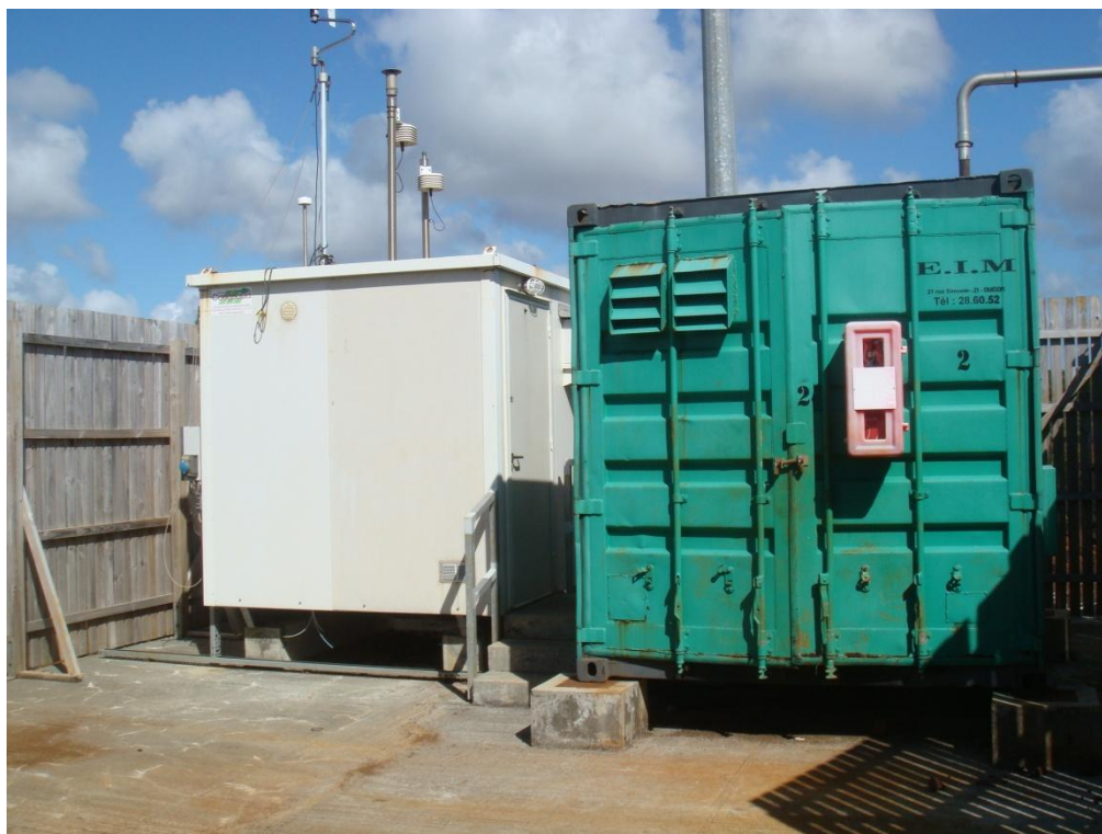
Figure 2: Station de Port Boisé
